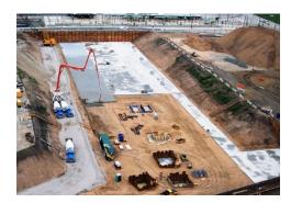
Here's a closer, but still too distant, shot of work on the mud slab. Notice the machine at the bottom center of the photo. It uses the same GPS technology that the bulldozer used to ensure exact elevations.
