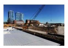
Construction workers apply a waterproof membrane over a concrete slab poured for a "bus box" Friday at Union Station. (Andy Cross, The Denver Post )The group developing Union Station as an expanded transit hub for RTD got a major boost Friday when the bond-ratings agency Fitch assigned an "A" rating to a key component of the project's debt.
