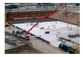
Now for the light rail station. This part of the project is far less dramatic in scope than the bus terminal, but vital nonetheless. The following photo is from the Millennium Bridge and shows that the station foundations are now approaching the Union Gateway Bridge (in the background). The ground surface will be raised to the tops of the concrete foundations/walls. Then the tracks can be laid, and the passenger platform can be built.
