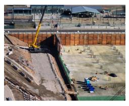
In the first photo above, you can see that six sections of the floor have been poured, bringing the total to date to about 7,000 cubic yards of concrete. The seventh pour is in progress right now. As you see in the second photo above, the first two forms for the concrete walls were put in place on Thursday afternoon and more may be added today. Assembled forms are laying along the side of the hole. It seems to take a few days to build one form but only a few hours to install it.
