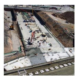
Here is a shot from the light rail station on Wewatta Street showing progress on the bus terminal walls. Eleven, 50 foot sections have been poured so far. As I mentioned previously, the wall is 19 feet high and two feet thick.
