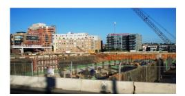
A new development today is the start of the plenum wall inside the bus terminal. In the center of the photo below, you can see the first form for that wall being placed to the left of the new, outside wall. The plenum is the conduit through which bus exhaust will be evacuated to the outdoors. I like to think of the process as exhausting the exhaust.
