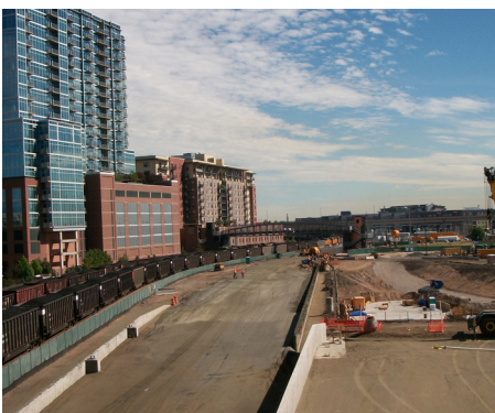
West edge of construction site showing the construction of the LRT retaining wall (August 2010)
