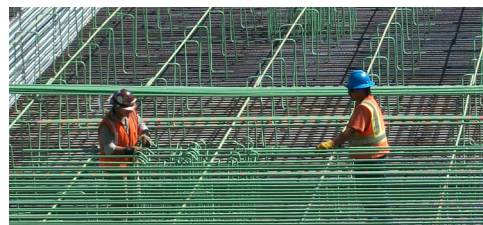
Tying rebar for four-foot thick concrete base of underground bus facility (August 2010)
