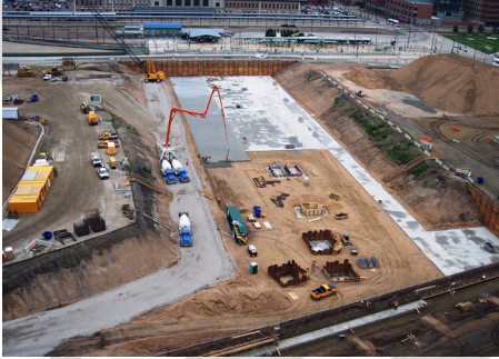
Underground bus facility "mud slab" pour in progress (July 2010, Rick Anstey)
