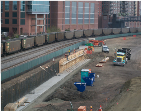
Construction of retaining walls for LRT (April 2010)
