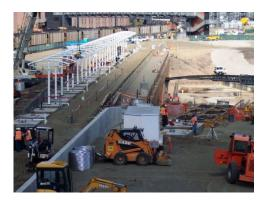
Second, there are several points of interest in the photo below. The walls of the bus terminal appear to be at least 75% complete; the plenum wall is about 30% done; and some of the columns inside the bus terminal to the left of the photo-center are now concrete instead of rebar. You have to wonder when they will place the first roof girder. Should we have a contest to pick the date?
