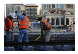
Workers fasten down the rails near the new light-rail station last week.
