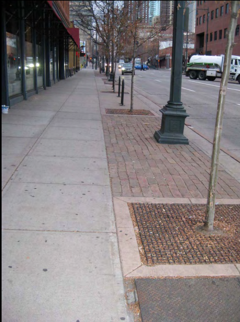
Granite and Brick
