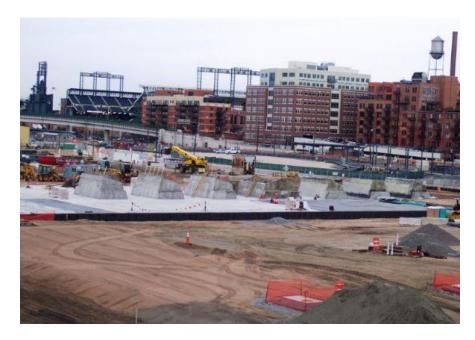
Here's a close-up shot showing progress of the bus terminal entrance/exit ramp. The floor of the ramp is complete and the walls are now being built.
