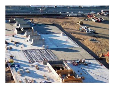
All seven skylights in the roof of the bus terminal have now been constructed and are visible in the following photo.
