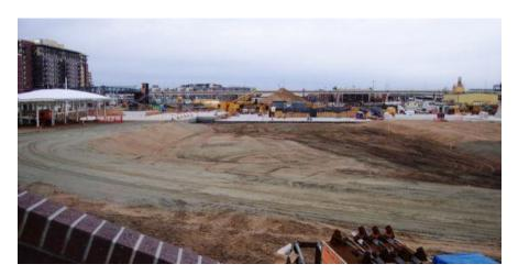
The next photo shows the first signs of backfilling dirt on the top of the bus terminal alongside Wewatta Street (top of the photo). Construction vehicles are now routinely driving across that part of the roof. You can also see that waterproofing material is being added to the center part of the roof that will carry Chestnut Place. Foundation and utility work for Chestnut Place has also been started on the 18th Street side of the bus terminal.
