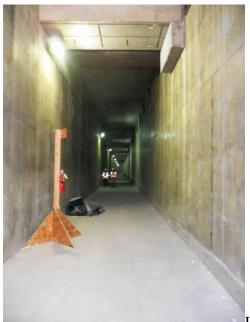
In the first photo *above*, look carefully at the plenum wall. You can see a series of rectangular holes along the top of it. In the first photo *below*, which I took from inside the plenum, notice the grates along the top. They fill the holes you saw in the other photo. Those holes/grates are the entry points into the plenum for the duct work. The second photo below shows the duct work between the beams in the ceiling of the bus travel lanes in the main part of the terminal.
