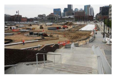
Now for the demolition. Looking closely at this photo below, you can see the top of an excavator in the hole where much of the passenger tunnel existed a few days ago. Part of the tunnel itself is visible to the right of the excavator's boom. The top of the ramp that led into the tunnel is clearly recognizable as a hole in the back of the station.
