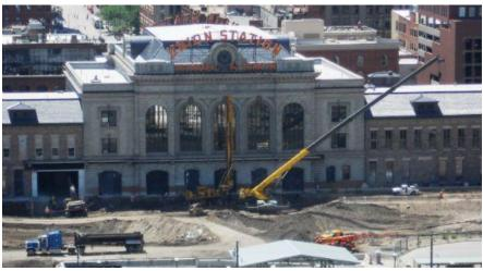
Speaking of protecting the station's foundation, think about the risks posed to the station by the heavy construction activity next to it. Kiewit is taking precautions to prevent damage to the old building including the installation of devices inside the building to monitor vibration levels.
