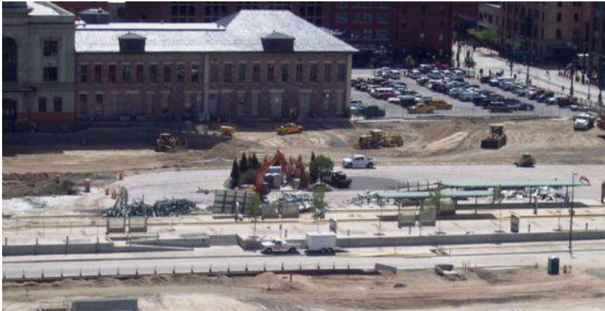
That conveyor system made relatively short work of moving dirt from the hole into huge piles along two sides of what is now the underground bus terminal. Digging for the second half of the terminal has been underway for a few weeks. Today, Kiewit started to assemble the conveyor system again (see the upper right corner in the photo below). This time, the dirt pile will be next to 16th Street where the tracks remain in the street.
