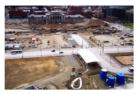
Almost all of the concrete that was the light rail station and mall shuttle station has been broken up, removed, and sent to the recycling location. Similarly, the top several feet of dirt that was contaminated by a century of coal dust is being removed from the site.
