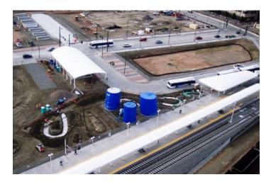
And what's up with the blue shrink-wrap on the new vent tubes? Well, there is a lot of work going on in the immediate area so the blue wrap is simply to protect them from damage.
