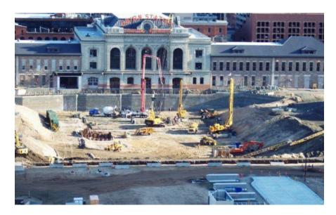
The pieces of equipment in the photo above are building caissons for the train bridges that will be part of the roof of the bus terminal. (I had to look up the definition of a caisson.) There will be eight sets of tracks (Amtrak, Ski Train, commuter rail) requiring four bridges. As we know, trains can be pretty heavy so the bridges will require deep, sturdy foundations. Therefore, the caissons.
