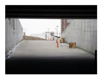
Exhaust is a very important aspect of this project since this is underground. Vents will open up leading exhaust through this hallway and out the vents by the light-rail platform. It will also be 'scrubbed' so the exhaust coming out of the vents will be odorless and colorless. How does fresh air get down into the bus facility? Easy! There is an air intake vent, pictured below. This will help keep fresh air in the bus terminal at all times.
