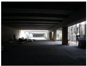
Here is where the phases of the terminal differ. Here we are looking at the commuter rail platforms from below. You can see the supports to hold the trains are much larger than the supports used for the bus terminal. Once enclosed, it will look uniform between both halves of the terminal.
