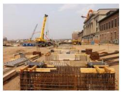
Below you will see another set of foundations being set for the trusses of the canopy. Needless to say, this thing is going to be massive. It stretches all the way down to the very north tip of the historic building and almost an entire city block west. I also took a picture of how large the anchors are going to be for these trusses. Impressive!
