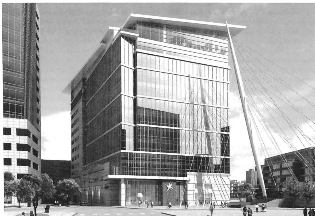
A rendering of DaVita world headquarters. The white cable-stayed bridge will allow pedestrians to cross an interstate highway.
