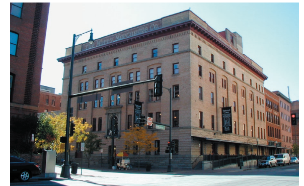
Adaptive reuse in LoDo with first three floors retail (Tattered Cover Bookstore) and residential lofts above.
