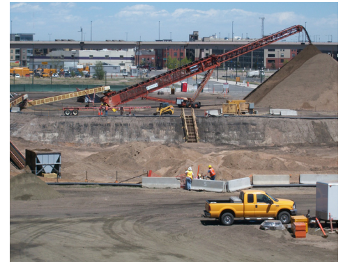
Conveyor system removing dirt from excavation into piles. May 2010.
