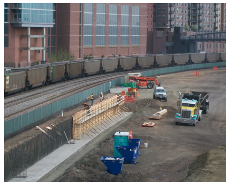
Construction of retaining walls for LRT. April 2010.
