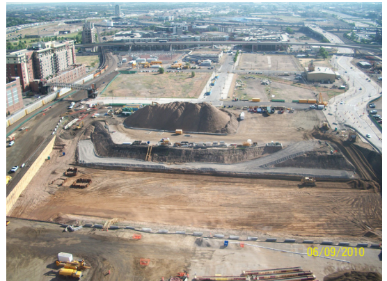
Western end of excavation for underground bus facility and dirt that will be used to backfill the excavation when structure complete. June 2010
